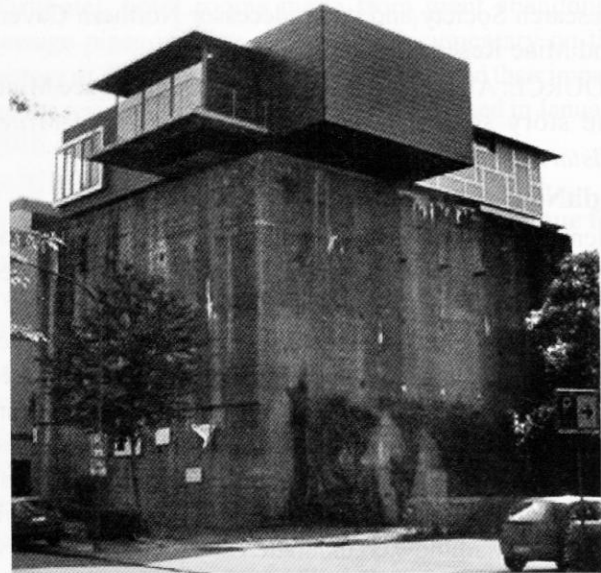
Completed Bremen bunker conversion
